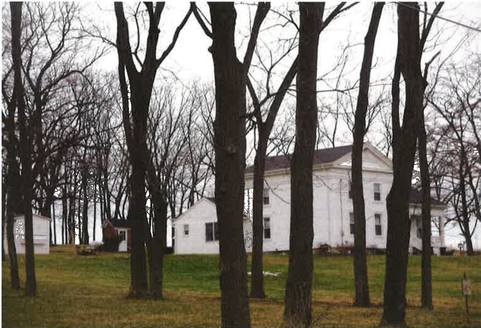
VIEW OF SUBJECT SITE
