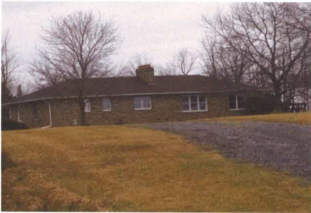
CLOSE-UP VIEW OF MAIN HOUSE - NORTH SIDE OF NEW BOSTON ROAD
