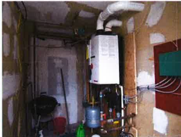
Utility room on rear of home
