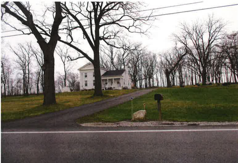
VIEW OF SUBJECT SITE
